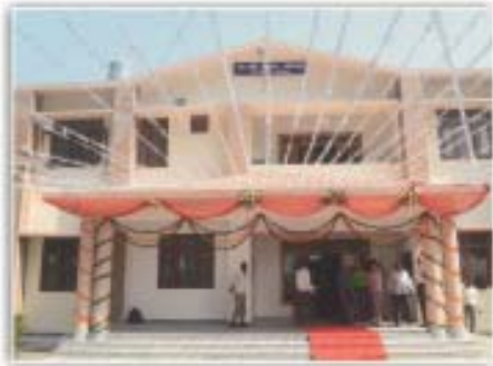
Building of ADR Centre at District Court, Haridwar
